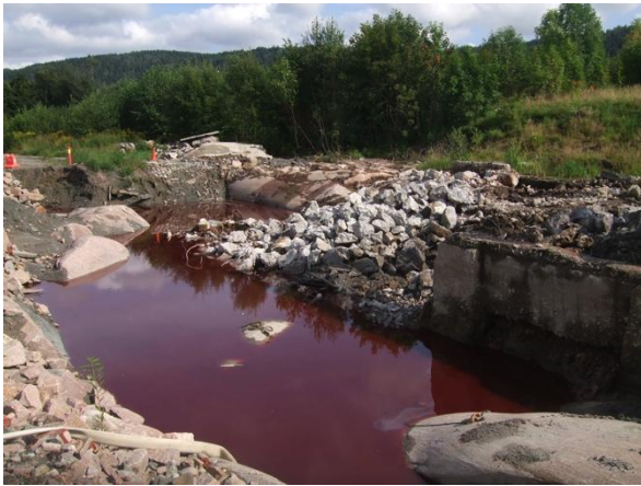
The foundations of the TNT building start to fall!
