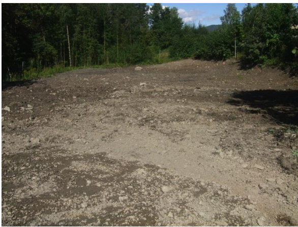
Internal land fill is refilled...finished!
